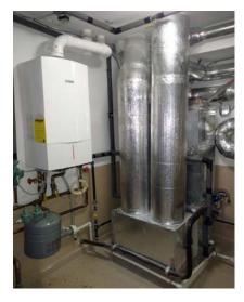
Solar thermal panels and a highefficiency boiler provide hot water for the hydrocoil heating system, while an ERV provides fresh air ventilation.
